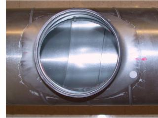
Fig. 3. Hole Cut in Duct with Neck Piece.
